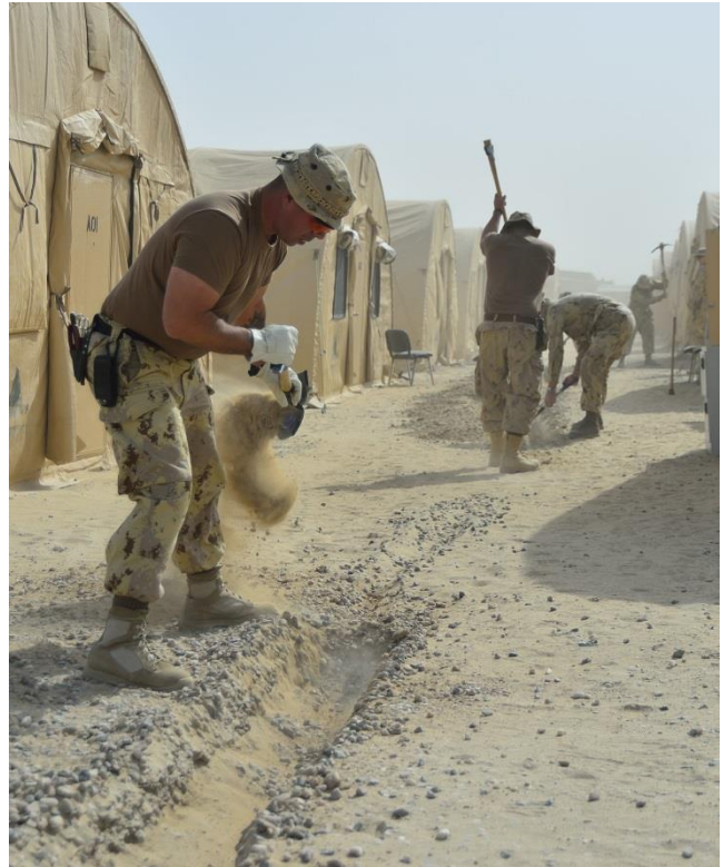
Figure 2-4: Digging trenches for communications conduits
